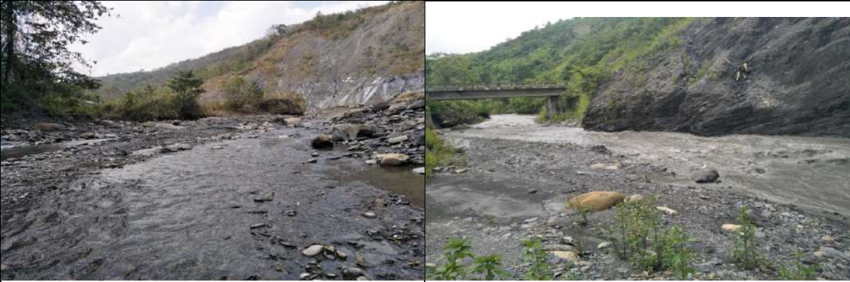
Photograph of station 4
