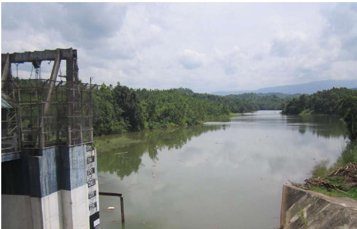
PLATE 3: STATION 2 KYRDEMKULAI DAM (EAST KHASI HILL, RI BHOI DISTRICT, MAGHALYA)
